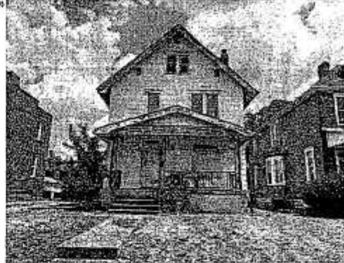
Vacant structure not boarded to code.
